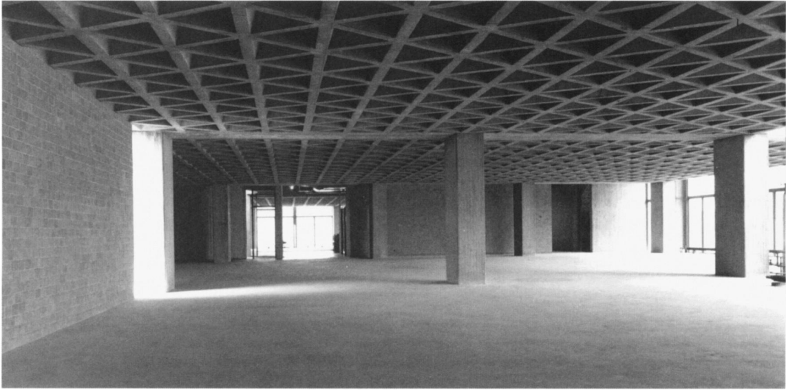
2 View of the interior before the installation of partitions.
