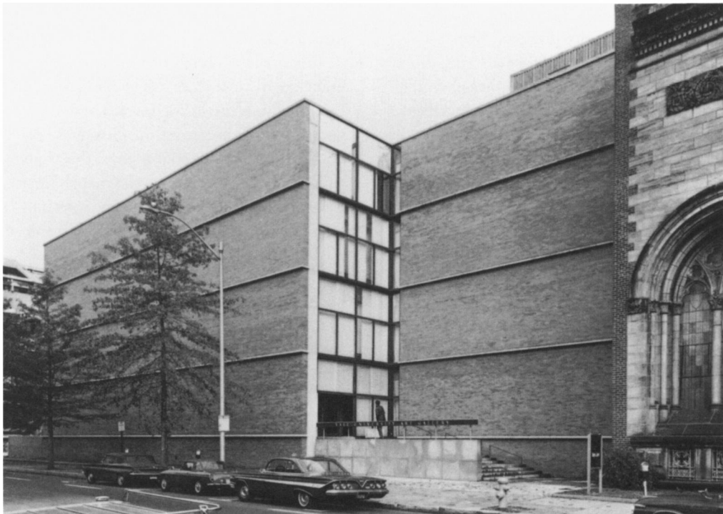
7 View of the building from Chapel Street.
